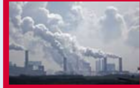
Fluorides, chlorine, sulphur, carbon monoxide
