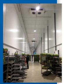
Dual discharge Güntner DUAL Vario DGN coolers with slowly rotating fans effectively prevent the danger of product dehydration in the corridors and production rooms as the coolers ensure draught-free air distribution.
