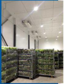
Güntner AGRI Application GACA coolers with blow-through fans and deflectors provide a very low dT inside the storage rooms. This ensures the dehumidification of the refrigerated goods is as low as possible.
