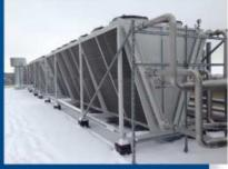
In winter, the whole waste heat of the compressors is used for heating, and during summer, the heat which is not needed is dissipated by means of a Güntner V-SHAPE Vario GVD condenser as well as three Güntner V-SHAPE Vario GFD fluid coolers/dry coolers
