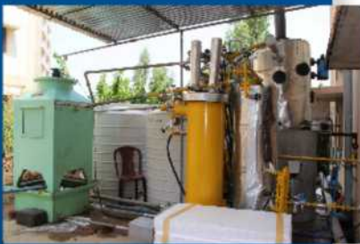
The small GreenCHILL cooling plant of the Indian New Leaf Dynamic company uses, among other things, the great amount of buffalo and cow dung available in India, other residues from forestry and agriculture and also biogas as primary fuel.
