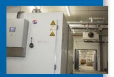
▲ Every cooler circulates up to 90,000 m<sup>3</sup> of air per hour and thus provides an ideal air distribution in the storage.
