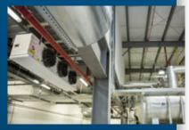
▲ The high external temperatures also require the air conditioning of technical premises and machine and staff rooms. The air coolers are supplied via the secondary water/glycol circuit  $(+8 \, ^{\circ}\text{C}/+16 \, ^{\circ}\text{C}).$
