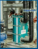
▲ Two thermowave TL 250 plate heat exchangers form the hydraulic interface between refrigerant and fluid.
