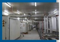
▲ 23 Güntner THERMOSTORE insulated unit coolers (flooded evaporators) registered for patent are installed above the picking area; they cool the storage rooms and the logistics facilities.
