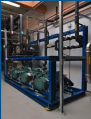
▲ CO<sub>2</sub> multi-compressor rack from the company Epta with heat recovery in the plant room.
