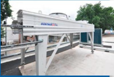
▲ Güntner Vario FLAT S-GVH gas coolers use small-diameter core tubes made of high-strength copper alloy. This substantially reduces the necessary tube volume to about 40 percent of that in typical stainless steel core tubes.
