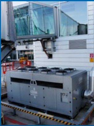
▲ The Güntner FLAT Vario unit is fully integrated into the PCA unit.
