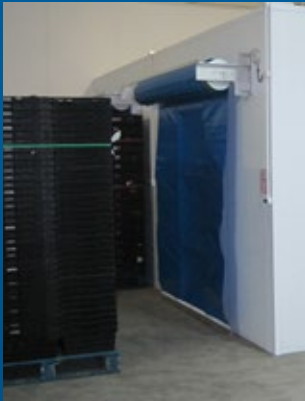
▲ In the cooling tunnel system at the site of the strawberry farmers, each one of the four cooling modules provides rapid post-harvest cooling to 10 pallets, around 3,400 kg per batch of fruit.
