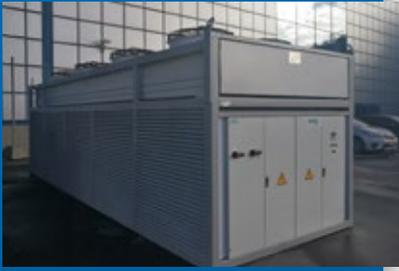
▲ The GCHV-type Güntner FLAT Vario condenser, together with the container solution, forms a structural unit named AIRCOOL monoblock.
