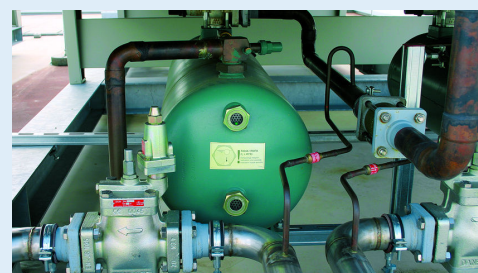
Liquid receiver with control and pressure absorber for controlling the condenser fans
