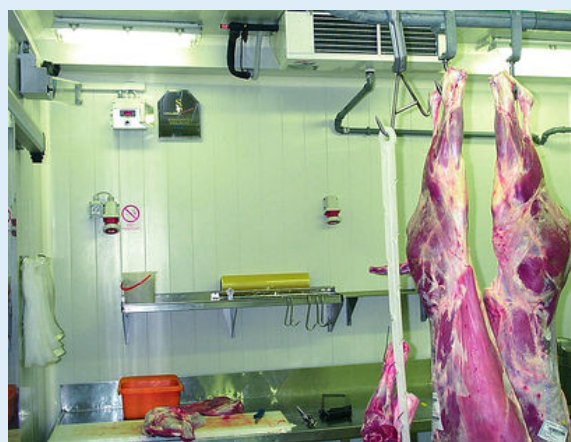
Draught-free working area cooling using the Güntner GDF evaporator
