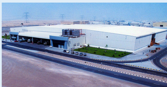
The large goods transshipment point with three stainless steel evaporative condensers on the roofed delivery zone
