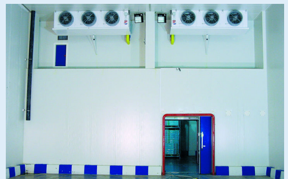
Two S-GHS 066D/38s at the dizzy height of around 8.5 m with maintenance gangway under the condensers
