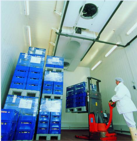
Güntner DHN with defrost flaps closed (evaporator in background obviously with excess warmth)
