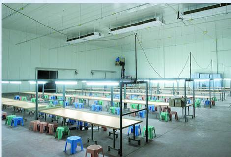
Type S-GBK processing room unit coolers: These ensure product quality in the consignment area. The units are specially developed for processing rooms, where they ensure quiet, draught-free airflow.
