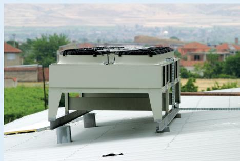
Güntner aircooled condenser (axial) GVH: Despite outside temperatures of 35 °C, Güntner condensers provide sufficient condensing capacity and Güntner evaporators maintain a relative humidity of 98 % indoors.
